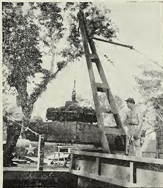
Hoisting an engine.
